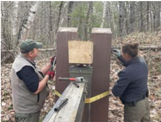
White and Rumaker repairing Togus Pond Gate
