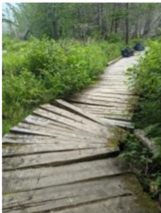
Sandy Stream Boardwalk before
