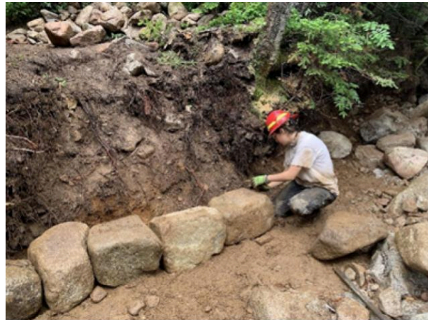
Upper Saddle Brook Bridge Retaining Wall
