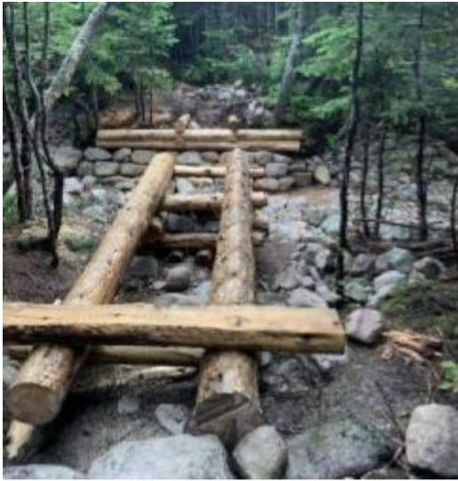
Upper Saddle Brook Bridge Replacement
