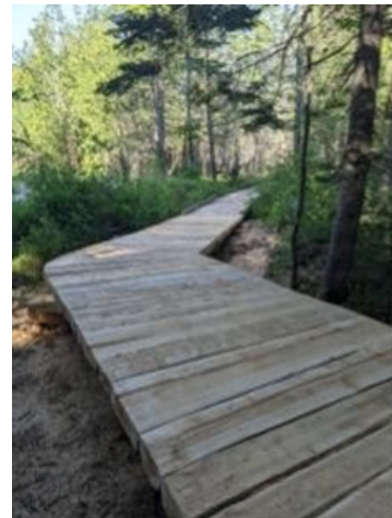
Sandy Stream boardwalk after
