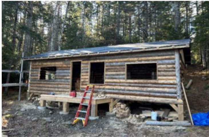
Daicey Pond Cabin 2, completely new construction
