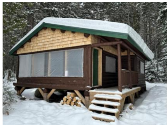
Daicey Pond Cabin 1 nearing completion
