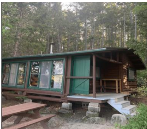
Daicey Pond Cabin 1 prior to renovations
