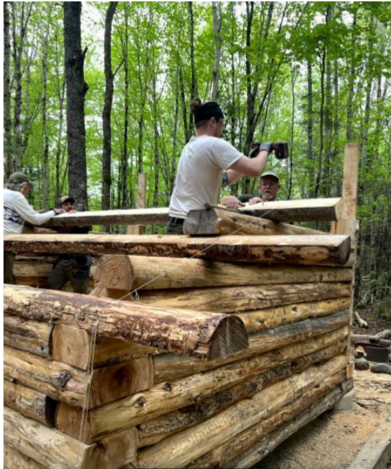
Rick Bray and BSP Staff building Lean-to 1 at Katahdin Stream
