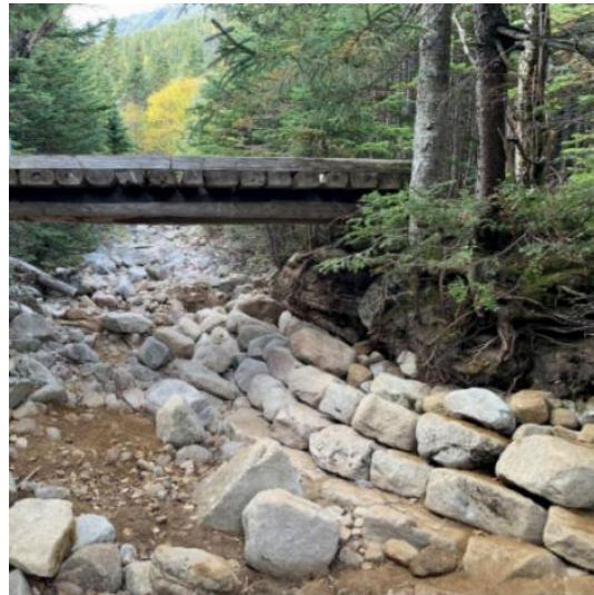
Upper Saddle Brook Bridge and armored streambank
