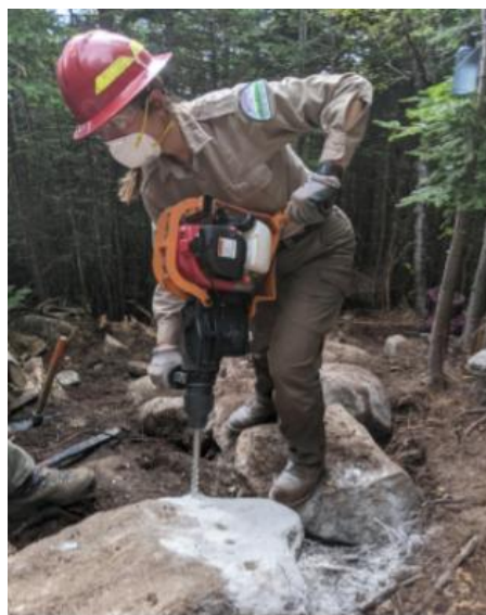
Mia Hayes drills & splits granite for Hunt Trail stone staircase project
