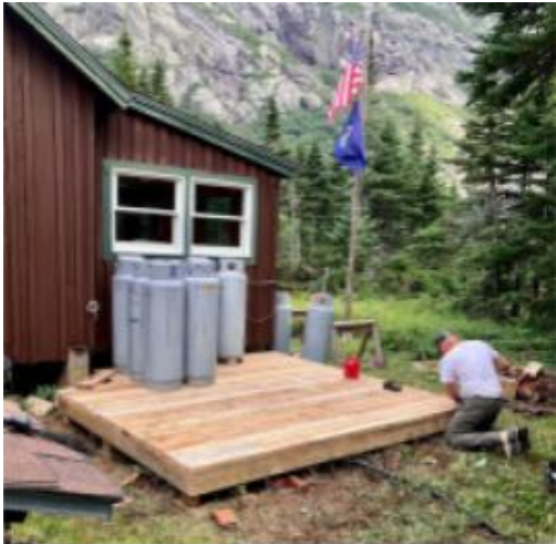
New Propane Platform, Chimney Pond
