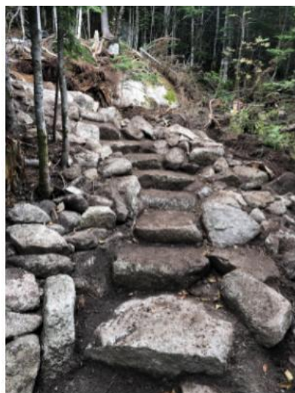
Hunt Trail Staircase
