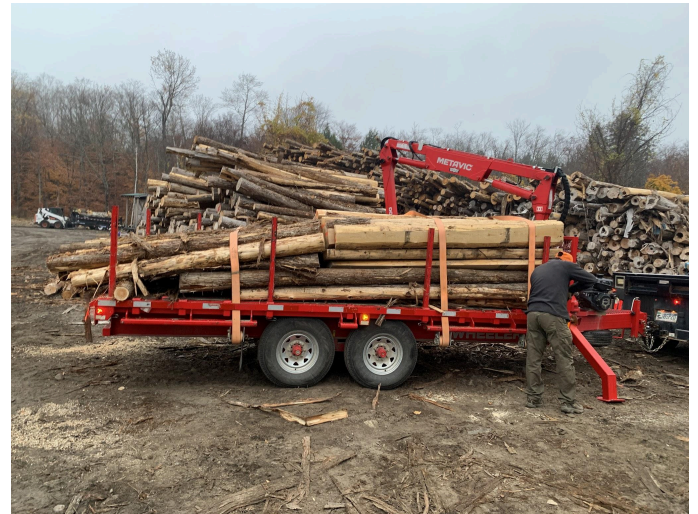
The first of many loads of bridge material
