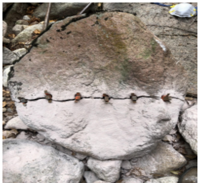
Figures 6. Crew Member Mia Hayes drills and splits granite for the stone staircase project.
