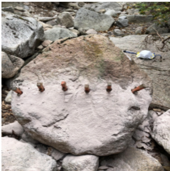
Figures 6. Crew Member Mia Hayes drills and splits granite for the stone staircase project.
