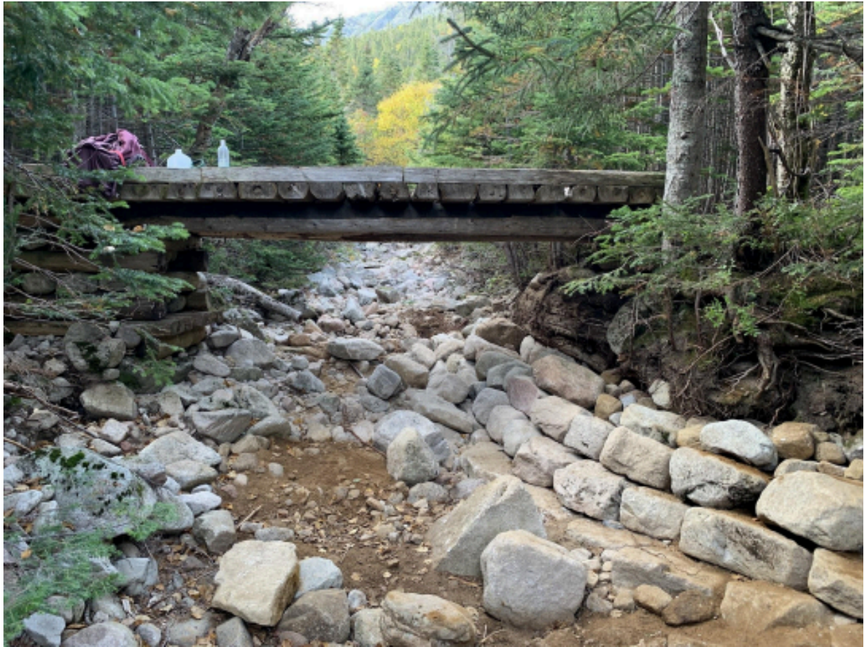
Figure 7. Upper Saddle Brook Bridge and the armored streambank
