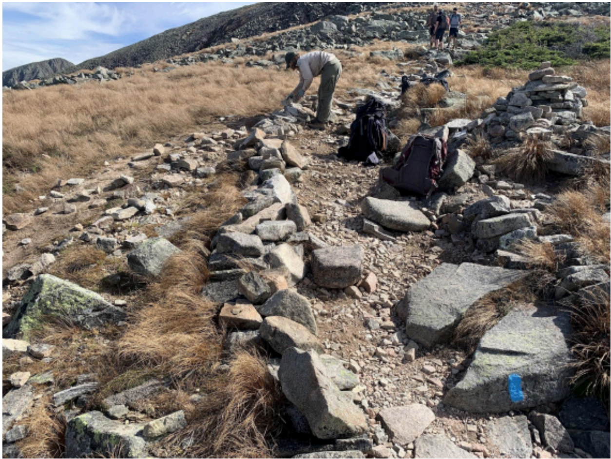
Figure 8. Crew Leader Emily builds a scree wall to delineate the trail and encourage hikers not to walk on the social trail seen to the left.
