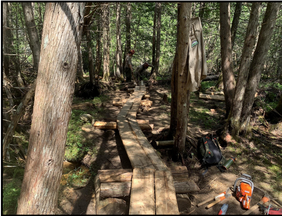
Approximately eighty feet of bog bridging was replaced adjacent to the elevated section pictured above
