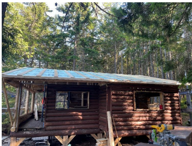
Cabin 1 side view with roof insulation and strapping
