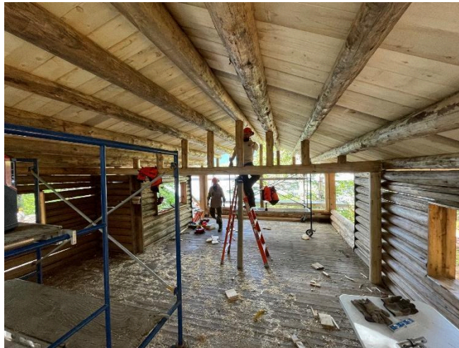
Cabin 1 interior with new roof purlins and sheathing
