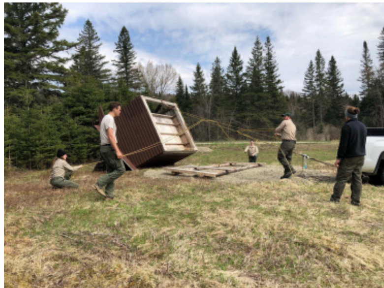
Figure 1. Trail Crew and Rovers use a compound 4-to-1 system to overturn the lean-to.
