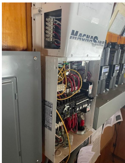
Making Wiring Adjustments to the Matagamon Solar Inverter/Charger
