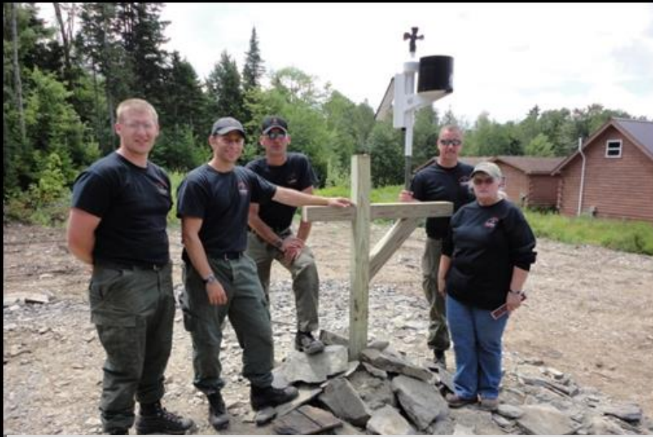
MFS Staff conducting station installation
