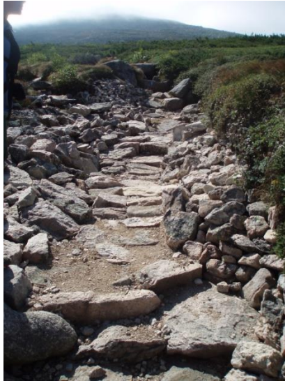
Figure 7-12 Step and stone work on the Saddle Trail
