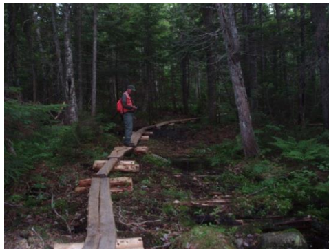
Figure 7-14 Bog bridging on the Katahdin Lake Trail
