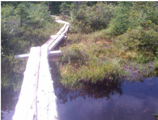
Installed bog bridging to access the Center Pond Lean-to (photo by M. Martin)
